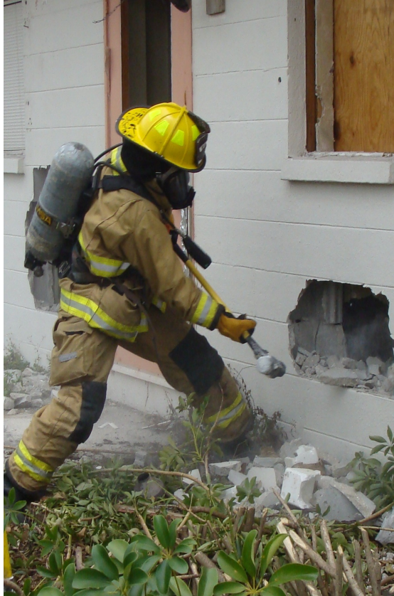
Firefighter Daniel Platas participating in training on breaching a cinderblock wall to gain entry into a home which otherwise is blocked from entry.
